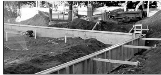
Construction of the new wading pool at Lake Hiawatha Park.
